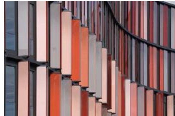
The Oval Offices in Cologne (arch. Sauerbruch and Hutton, 2010). Features vertical axis glazed sun louvers for light regulation (photo by M. Brzezicki).
