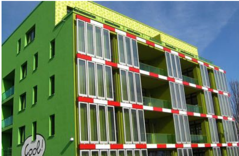
BIQ house', Hamburg, Germany. (Splitterwerk, Arup & Colt international). Features integrated microalgae which are used as bio-reactors inside panels.
